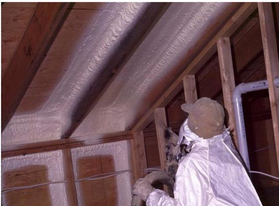
For flat ceilings, if recessed light fixtures are installed, do not spray polyurethane foam directly to the fixture; follow the fixture manufacturer's recommendations for insulation and/or venting the fixture. Some fixture types require that a gypsum board box be built around them prior to application.
