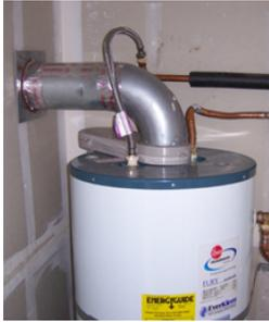
Figure 3: Direct Vent water heater. Sealed-combustion appliances are located close to an outside wall and vent through the wall. A double-walled vent tube functions as both air intake and exhaust flue. (No special requirements when air sealing building.)
