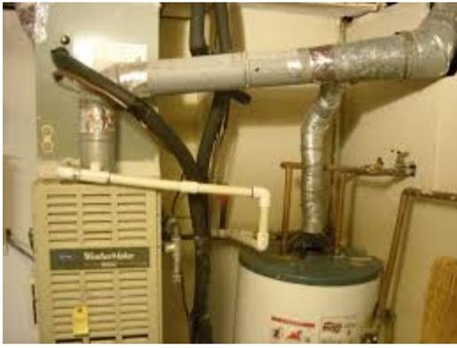
Figure 2: Typical open-combustion furnace co-vented with open-combustion water heater. (Requires fresh air source.)
