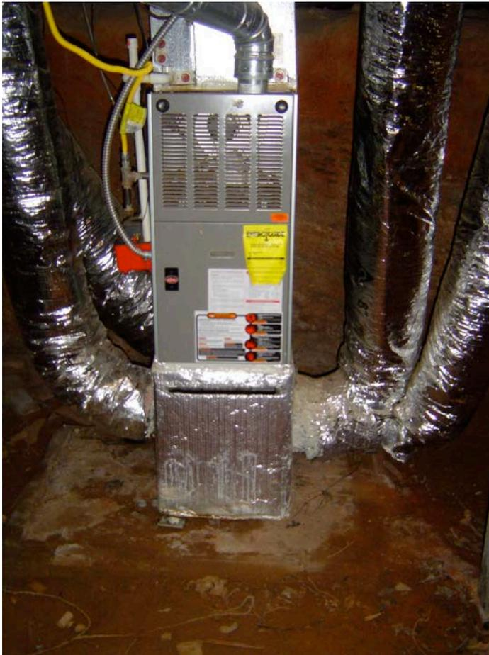
Figure 5: Draft fan-assisted HVAC system in a crawl space. The fan is designed to pull combustion by-products out of the heat exchanger and direct them into the exhaust flue. The fan does not propel the exhaust gases up the chimney; these appliances rely on the buoyancy of the hot exhaust to rise up the flue and vent out. This appliance is open-combustion and subject to the aforementioned considerations.
