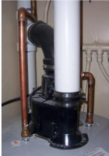
Figure 4: Powered vent on a water heater. Powered vents employ a blower to push exhaust gases out the exhaust vent pipe. Typically used for long vent runs. (No special requirements when air sealing building.)
