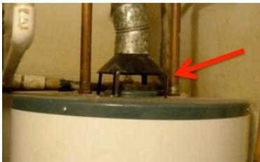
Figure 1: Typical open-combustion water heater. Arrow indicates the entrance to the exhaust flue.
